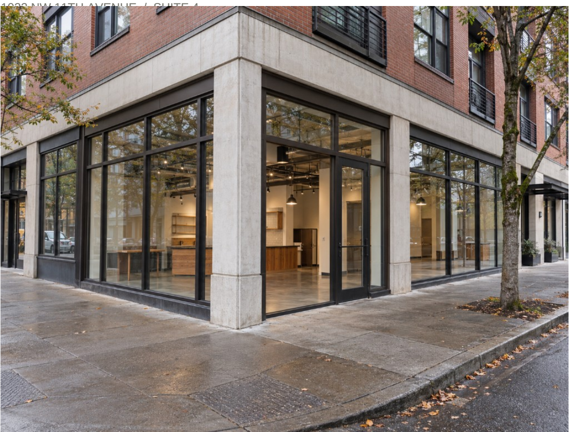
Existing visible condition / exterior storefront / does not establish use, dimensions, or compliance
